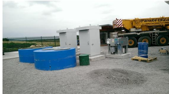
**Figure 11: Two modular Beacon FES systems installed in Ireland for Schwungrad Energy as a renewable / battery hybrid demonstration.**
